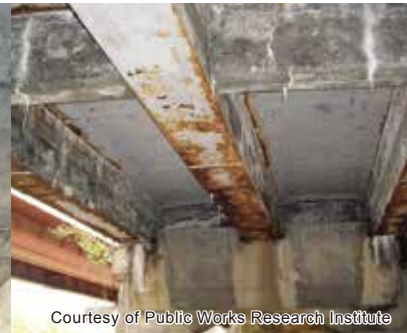
Courtesy of Public Works Research Institute
