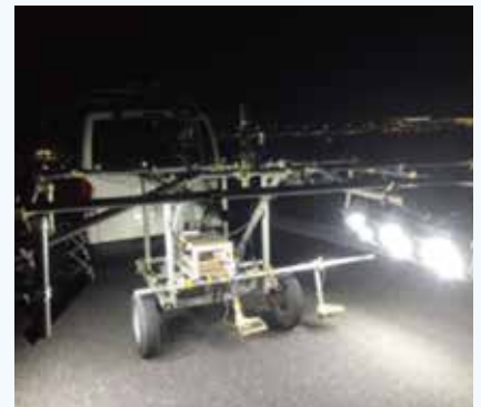
A monitoring site demonstration on the runway of an airport
